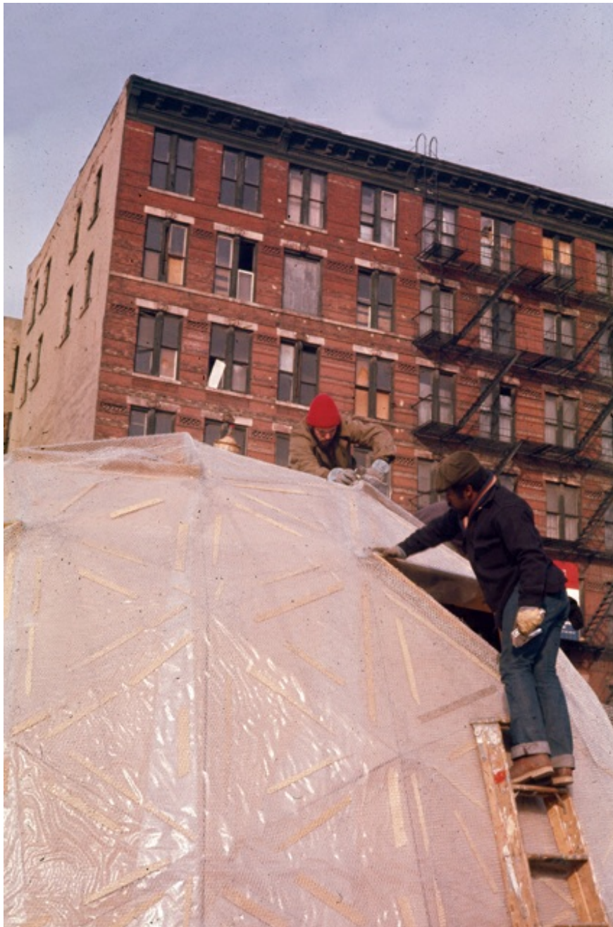
Construction on a geodesic dome.
